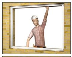
1. Place the frame on spacers into the wall opening.
